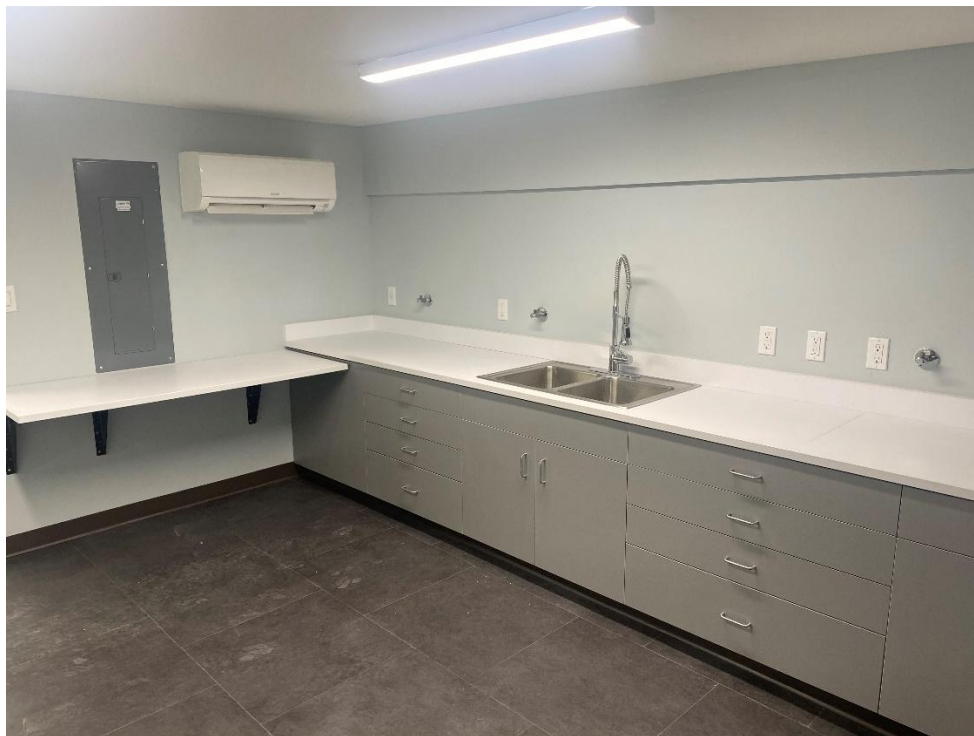
Work Area 2 - Cabinets with Sink (Basement)
