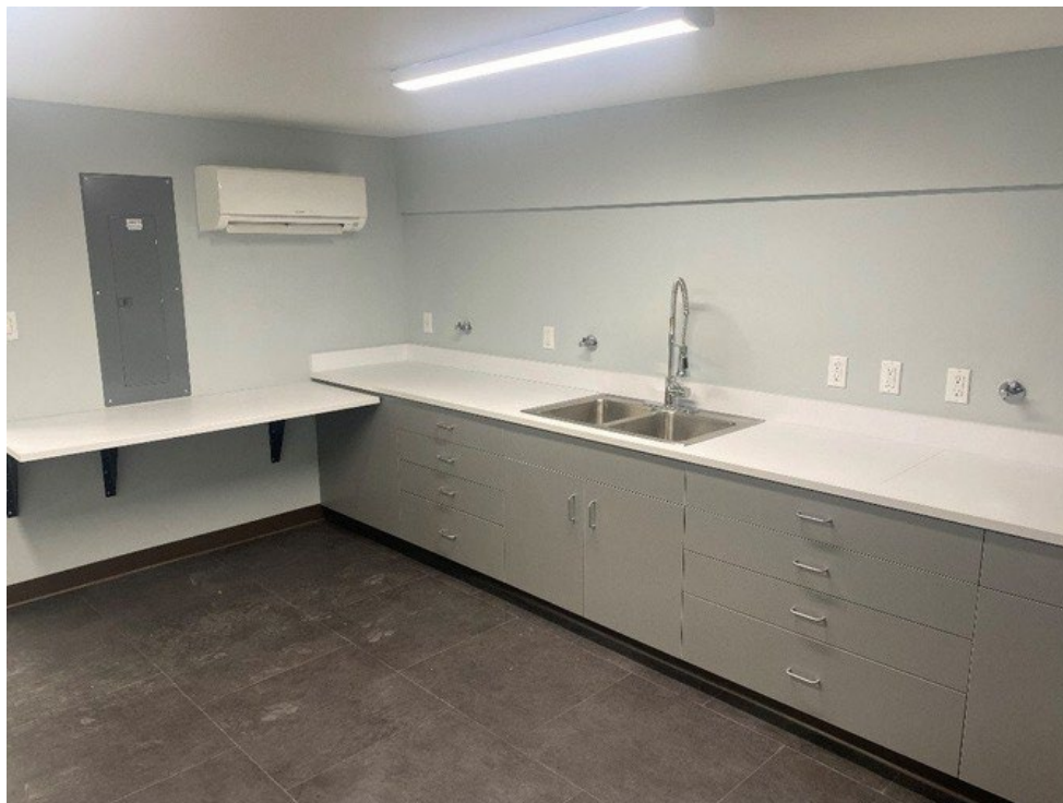
Work Area 2 - Cabinets with Sink (Basement)
